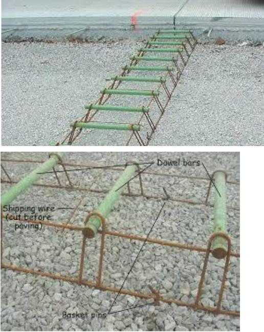
• Contraction & expansion joints are provided in rigid pavement due to temperature variation. (Increases or decreases)
