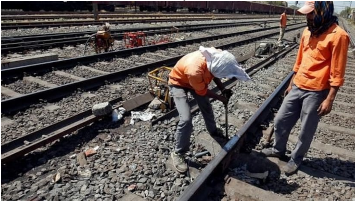
Track sleeper is under construction
